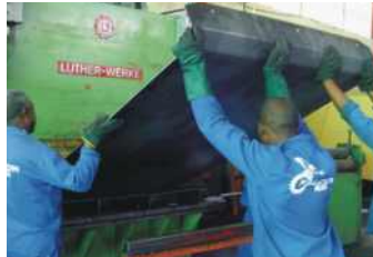
Bending Hull to 45 degrees
